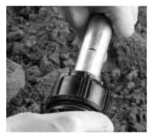
**4. Pipe Insertion**Insert the pipe fully into the fitting up to the witness mark.
